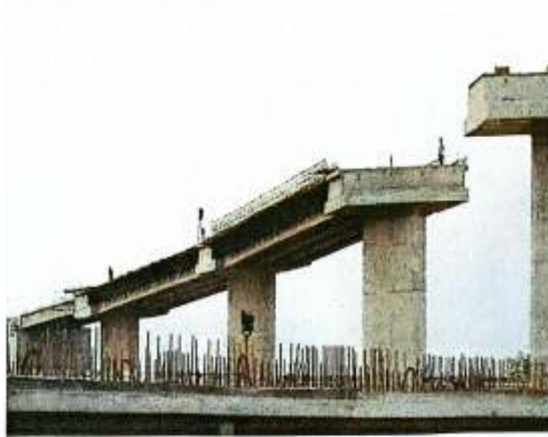
Gambar 2.5 Jembatan Beton Prategang
